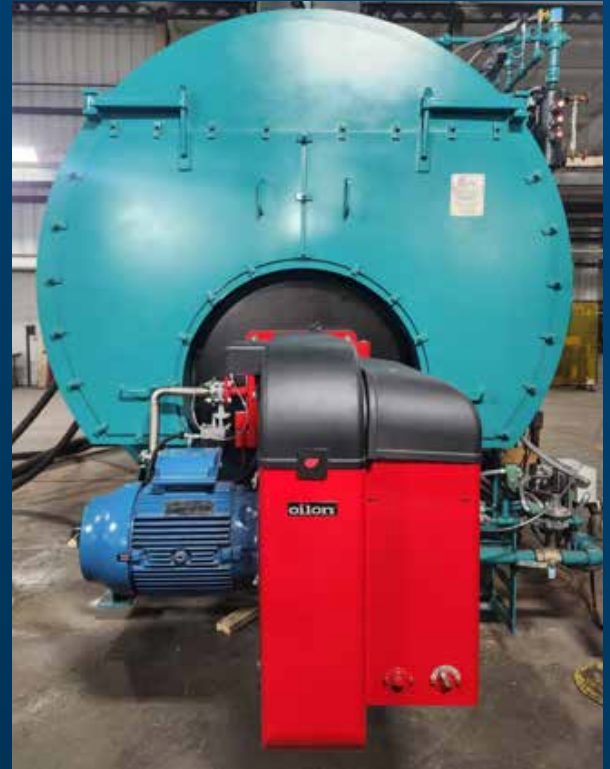
GP-600 M LN30, burner capacity 3 800 kW
