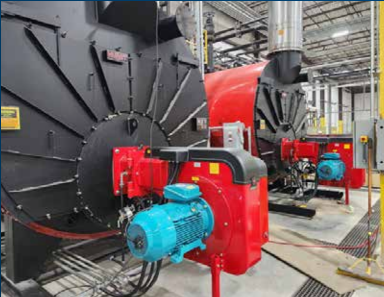
2 x GP-600 M-II LN30, burner capacity 5 400 kW
