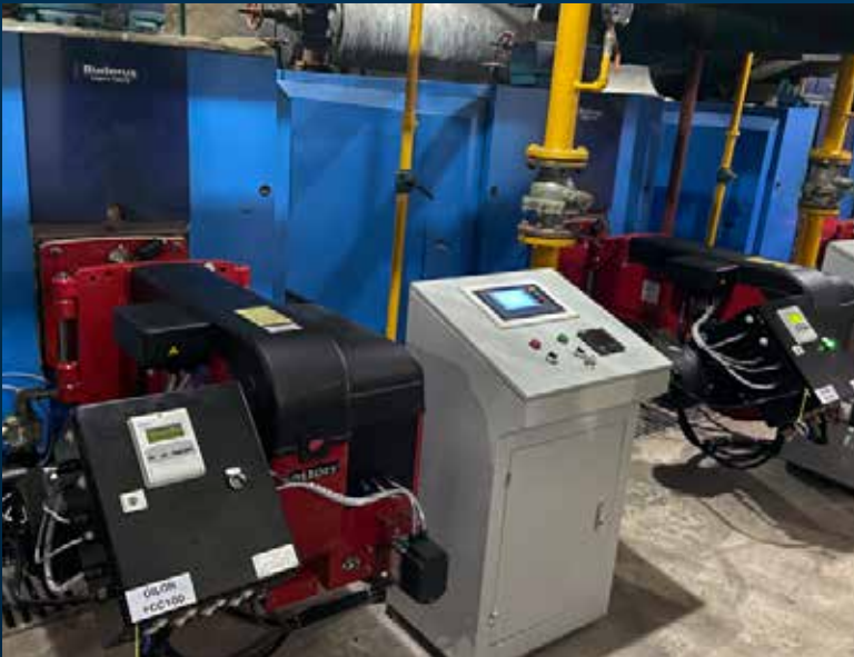
3 x GP-250 M LN30, burner capacity 1 400 kW
